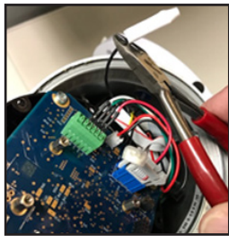
Cut the white insulator
